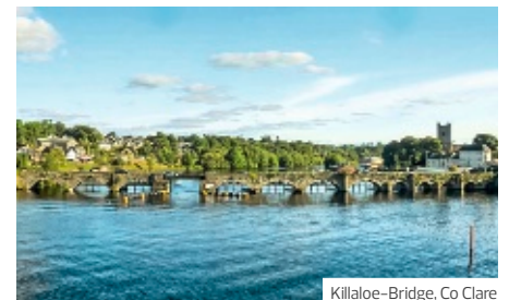
Killaloe-Bridge, Co Clare
